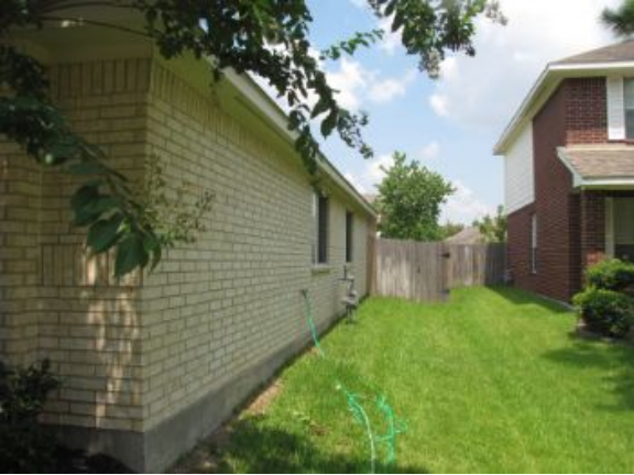
North Side of Home
