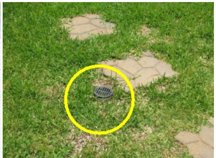
Drains installed in yard
