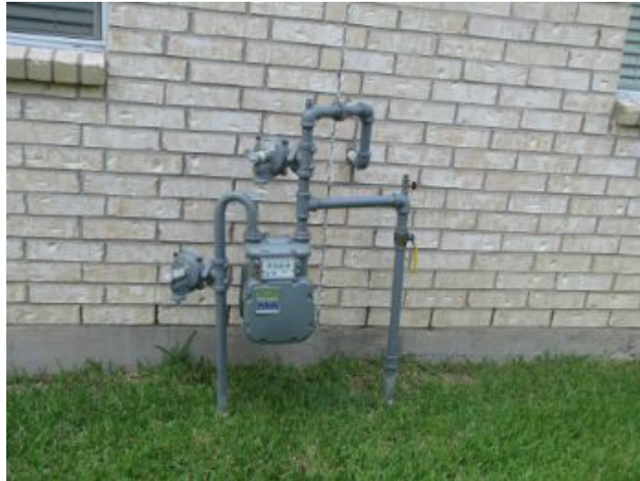
Gas meter - Checked for leaks - None detected.
