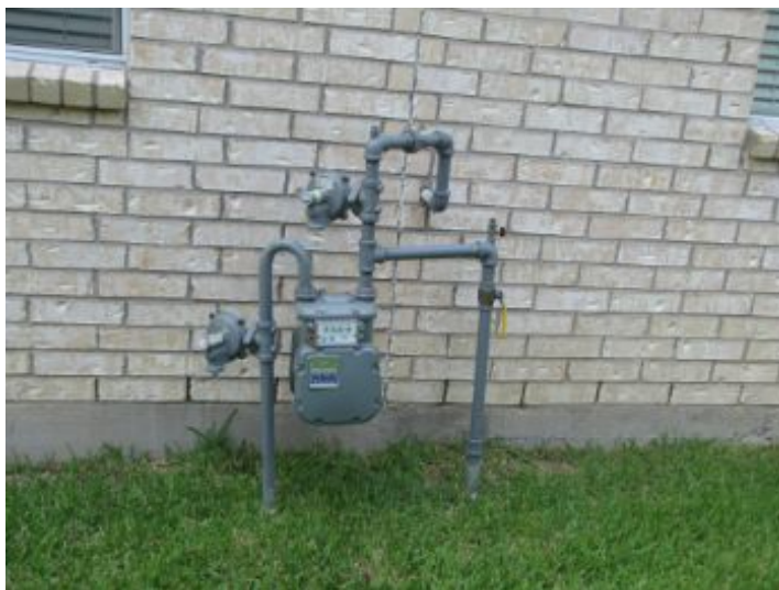
Gas meter - Checked for leaks - None detected.
