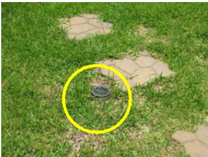
Drains installed in yard
